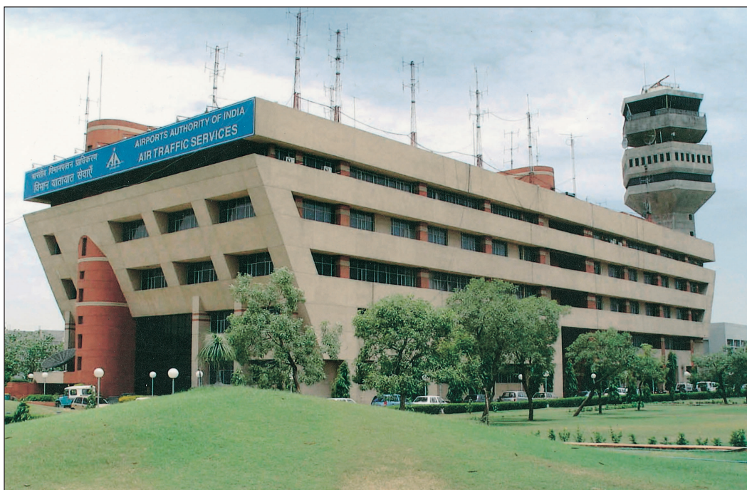
Air Traffic services, IGI Airport, New Delhi.
